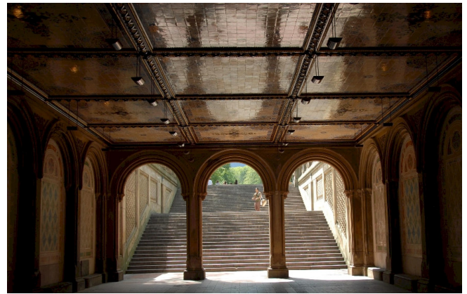
Pedestrian passageway, running beneath the 72nd St. Cross Drive, with Victorian Minton tiles, in 2007
