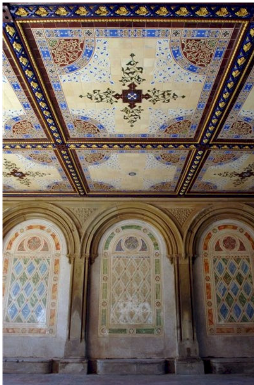
Ceiling Detail of one of the 49 tile compositions
