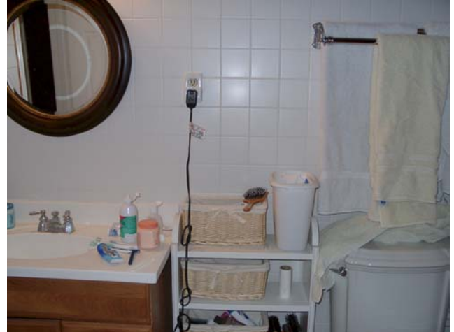
The bathroom - BEFORE
